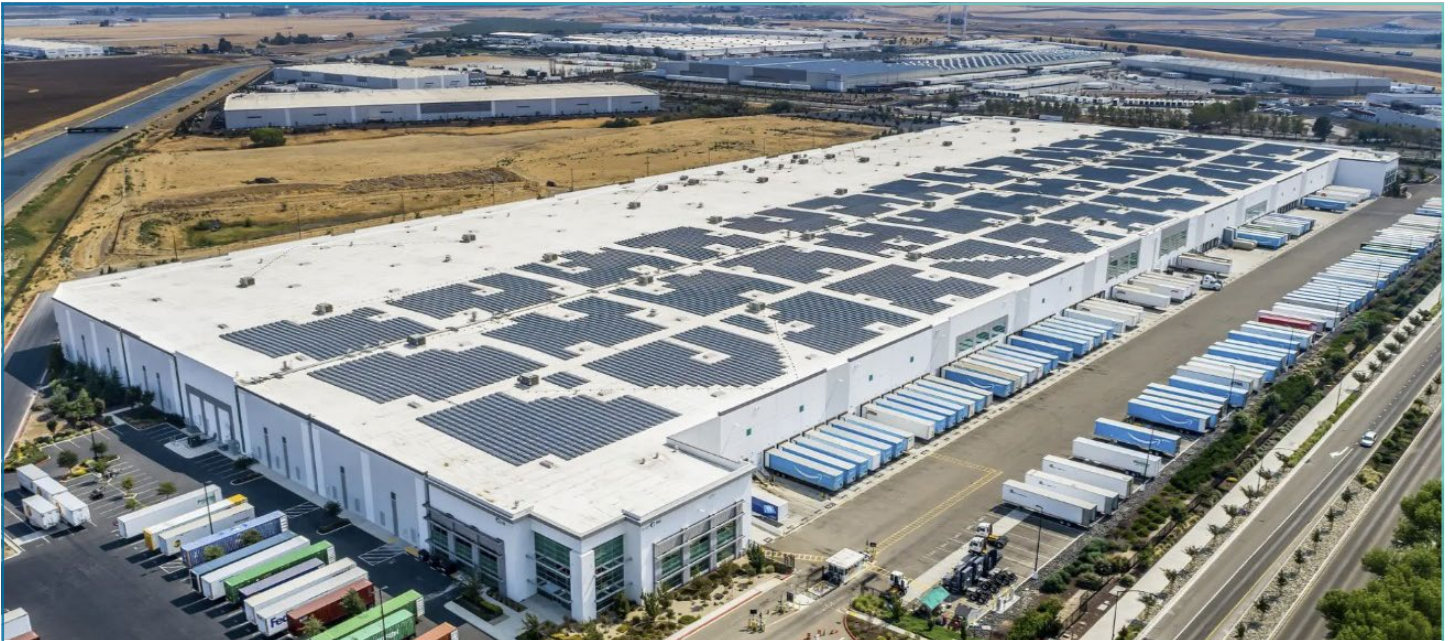
1M SF roof with smoke vents, no skylights and solar; skylights were removed to reduce heat gain
