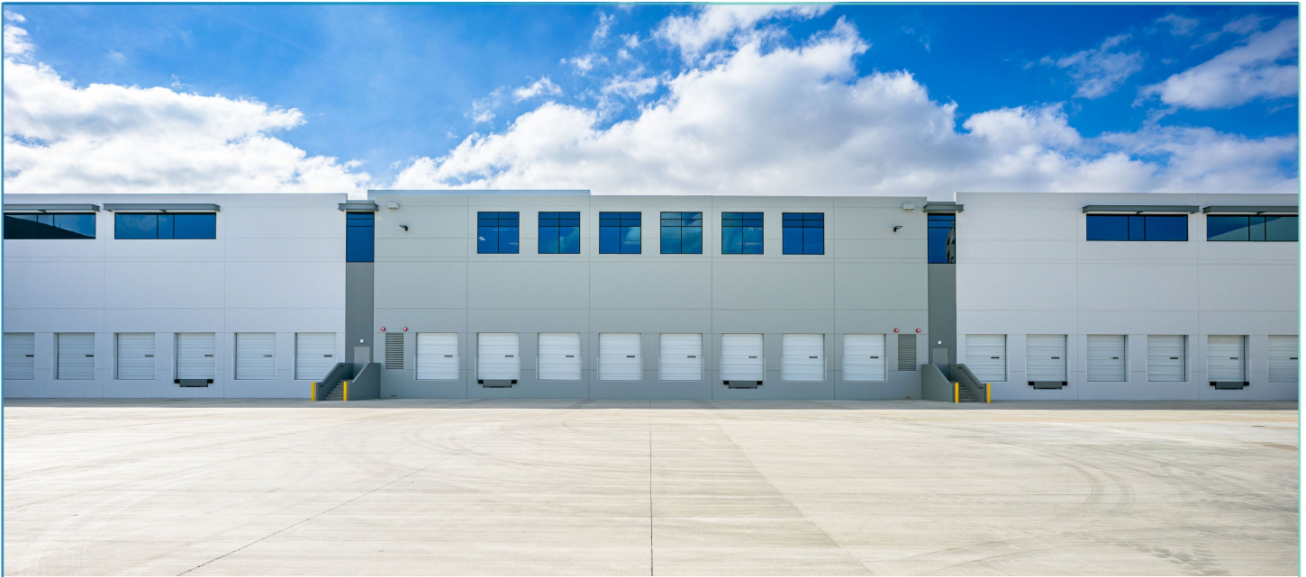
Clerestory windows above dock doors
